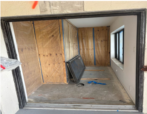
Figure 3: Bending/shearing and corrosion of aluminum track Unit 209; Unit will require new doors and windows at this bedroom location
