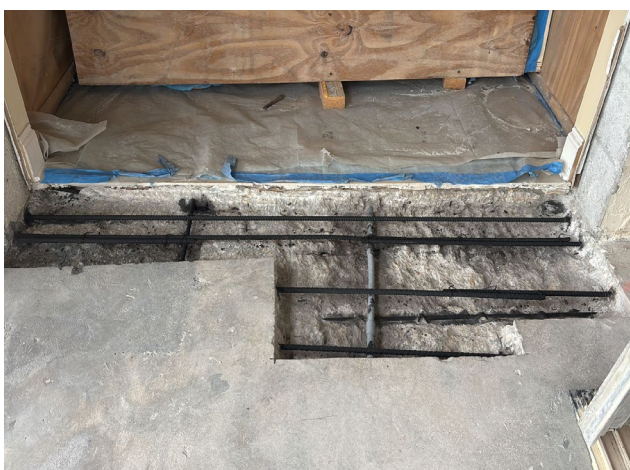
Figure 6: Unit 509 concrete placed back along the threshold on Thursday, 7/17
